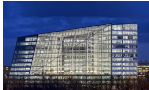
Figure 7: office connected lighting system in 2014
