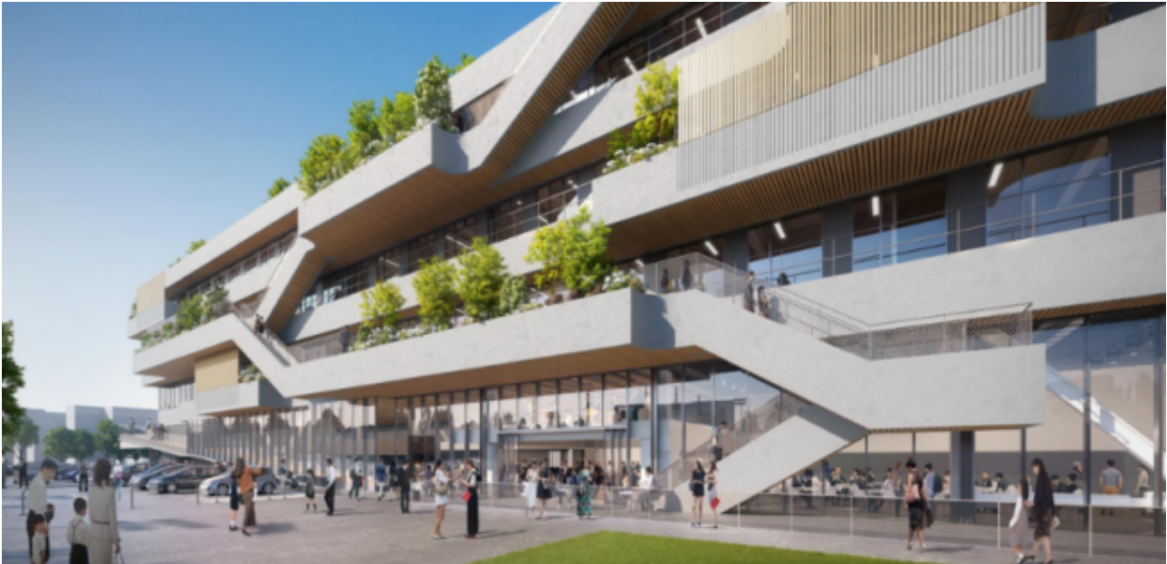
Figure 10 External view of the STATION Ai building
